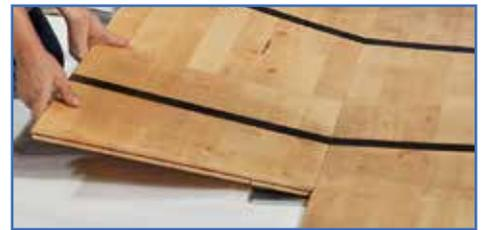
Each floor panel is easily locked into position by means of factory fitted metal brackets.
